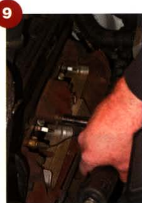
After pulling the plug wires off and out of the way, we removed the six bolts from the manifold. We ended up removing the plugs, too, just to be safe and check that they were clean.
