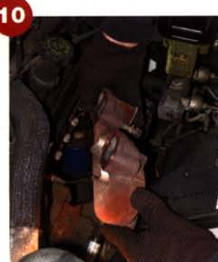
Now the manifold could be pulled out, allowing any debris left on the mounting surface of the head to be cleaned off.
